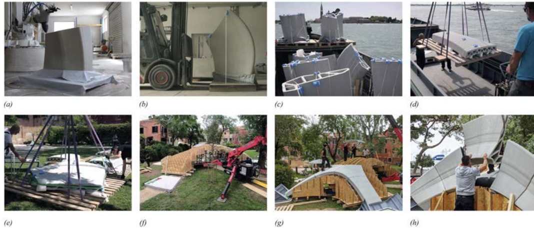
Figure 103 – Printing, construction, and assembly. (a) 3D printing of block. (b) Preparation for transportation. (c,d,e) Transportation and storage on site. (f) Erection of scaffold. (g) Placement of deck blocks. (h) Placement of key stone balustrade block.
